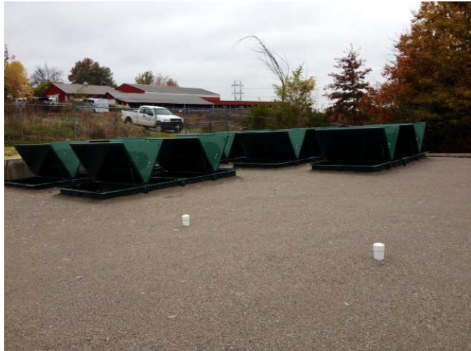
Figure 2: Replacement media installed at Red Rock WWTF in 2013
