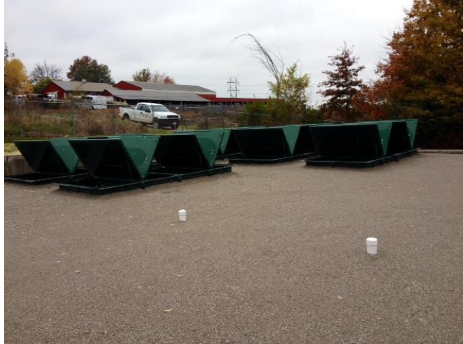
Figure 2: Red Rock WWTF
